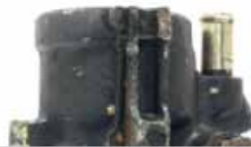
The mounting lug is broken
